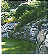
Planted retaining wall
